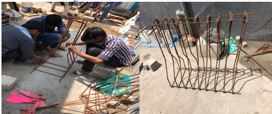
Figure 5.16 Reinforcement Detail
