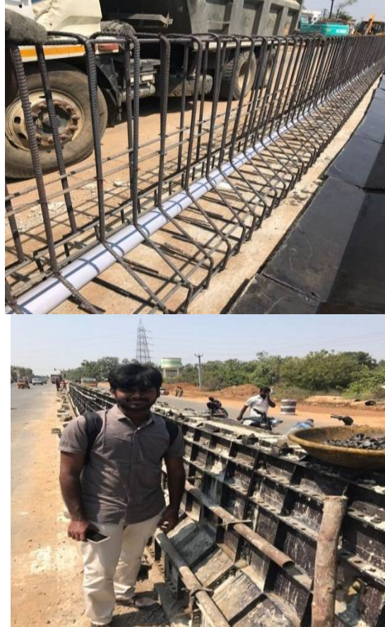
Figure 5.3 Construction of Concrete Barrier at Padapai
